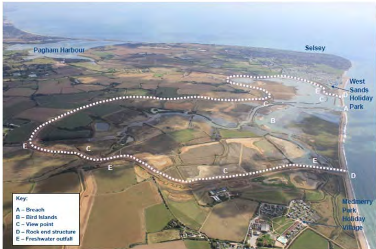
Figure 5 - Medmerry managed realignment scheme (ICE, 2015)
